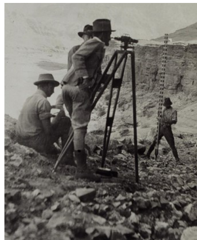
Photo 2: Leveling down the trail into Glen Canyon. Level party of Fred E. Joekel. Glen Canyon, Arizona. 1921.
